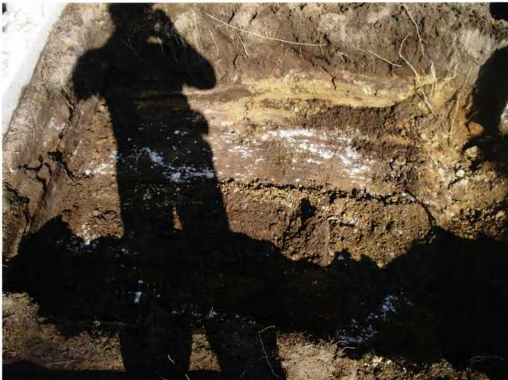
Picture 2: UST 318Ash excavation in progress.
